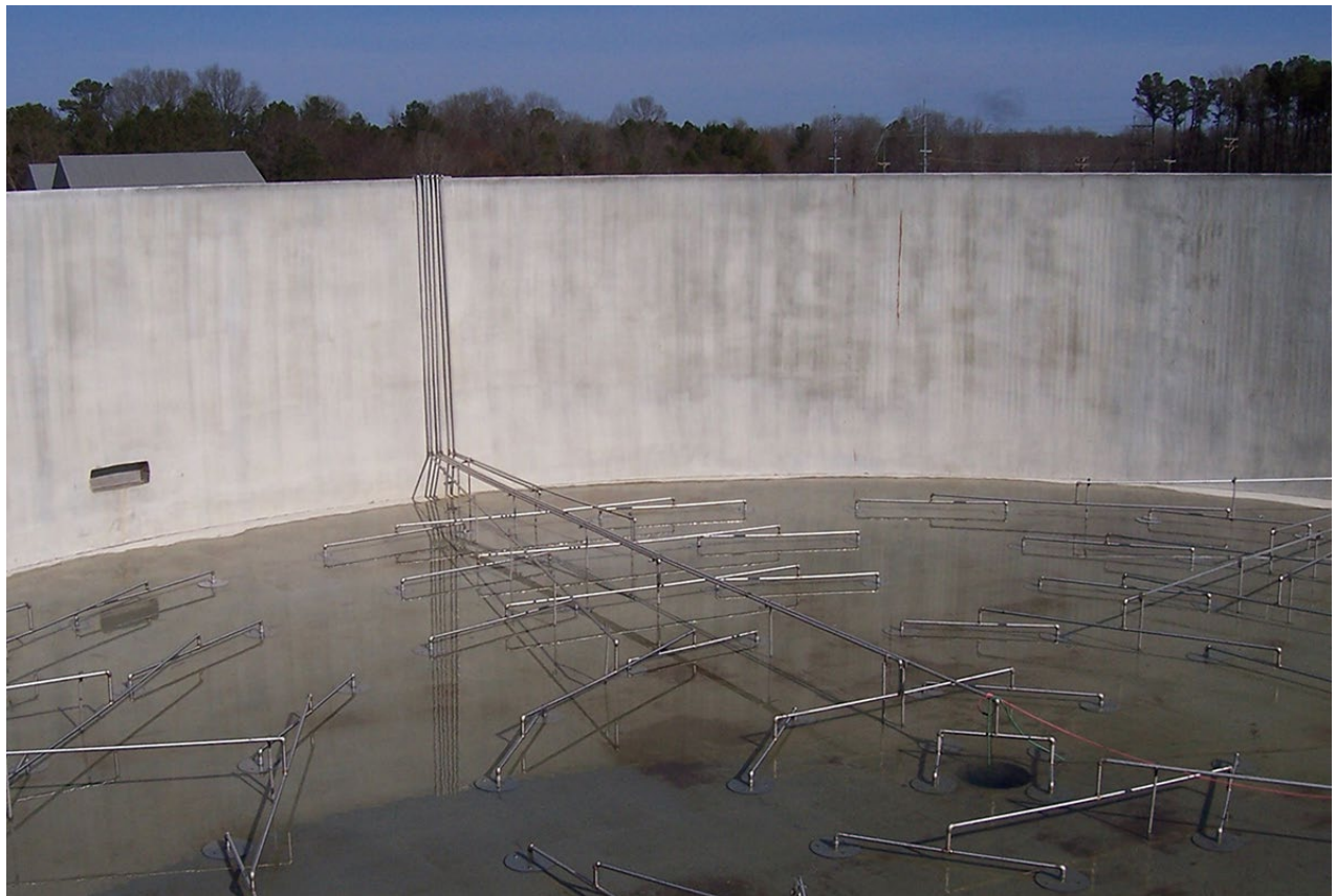
Example image of 120' diameter municipal wastewater sludge tank
