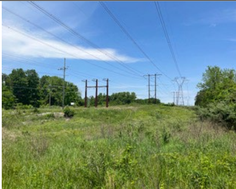
Photo #: 6 Photo Shows a View of: Existing Transmission Lines
