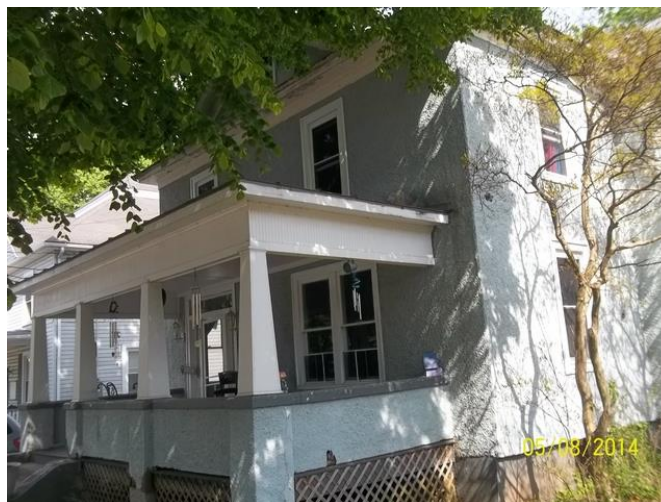
View of Side Elevation – 18 East Stonewall Drive
