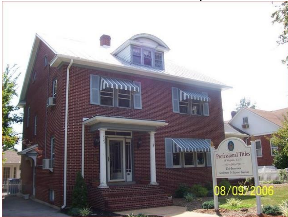
View of Front Elevation – 425 N. Royal Avenue
