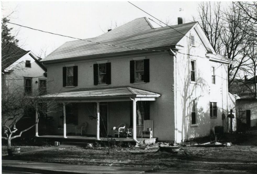
Photo 1 – view of front building elevation – historic district survey
