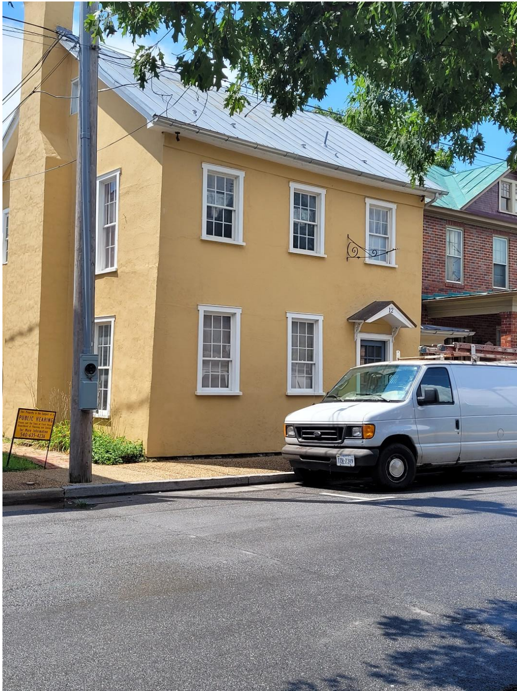
View of Front Elevation – 12 Chester Street
