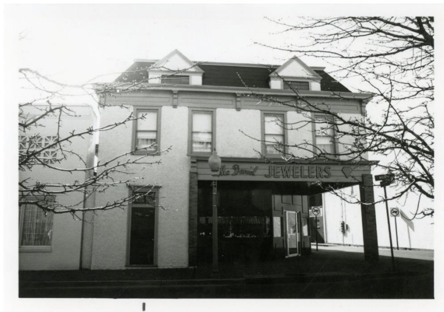
Photo 1 – view of front building elevation – historic district survey
