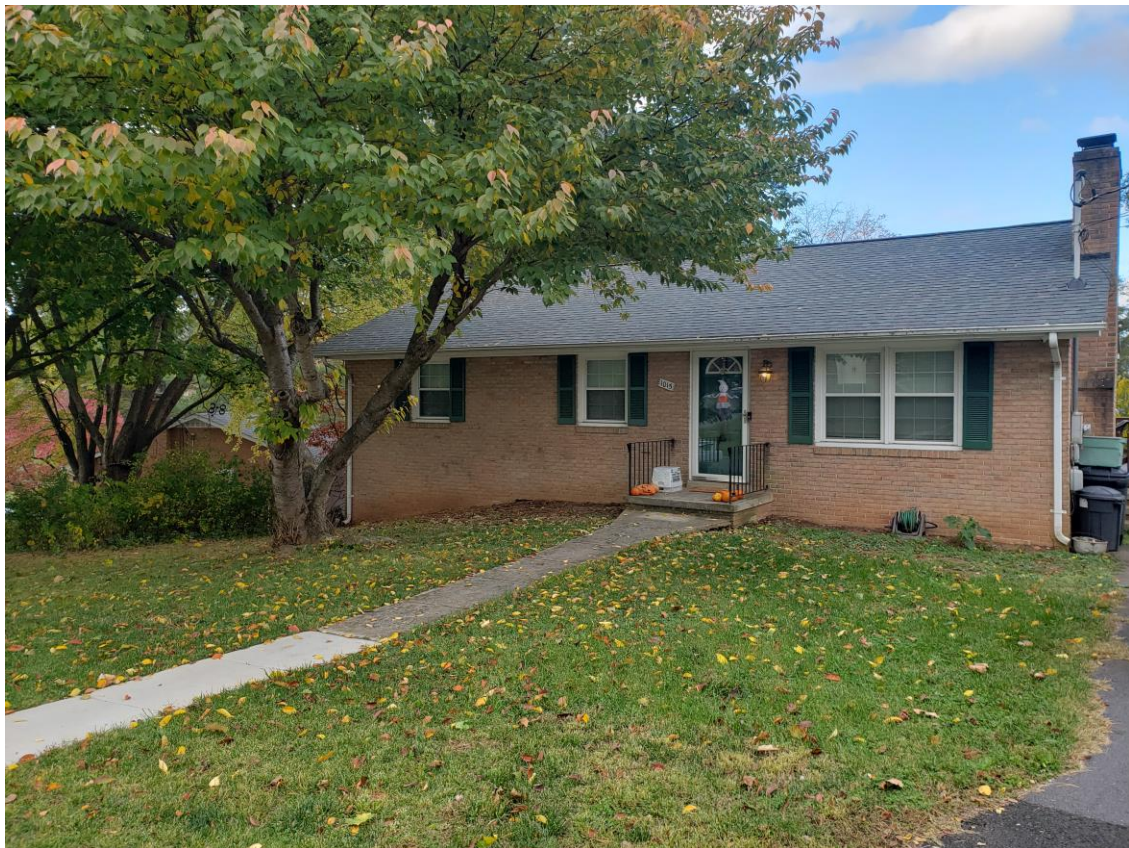
Front Elevation – 1015 Wine Street
