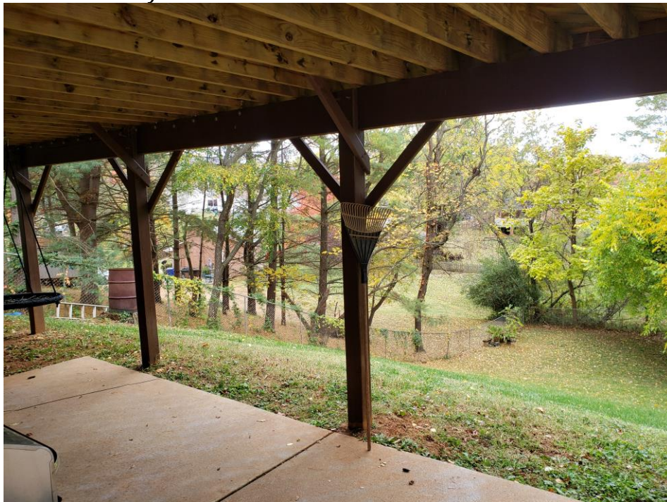
Right Rear Elevation – 1015 Wine Street
