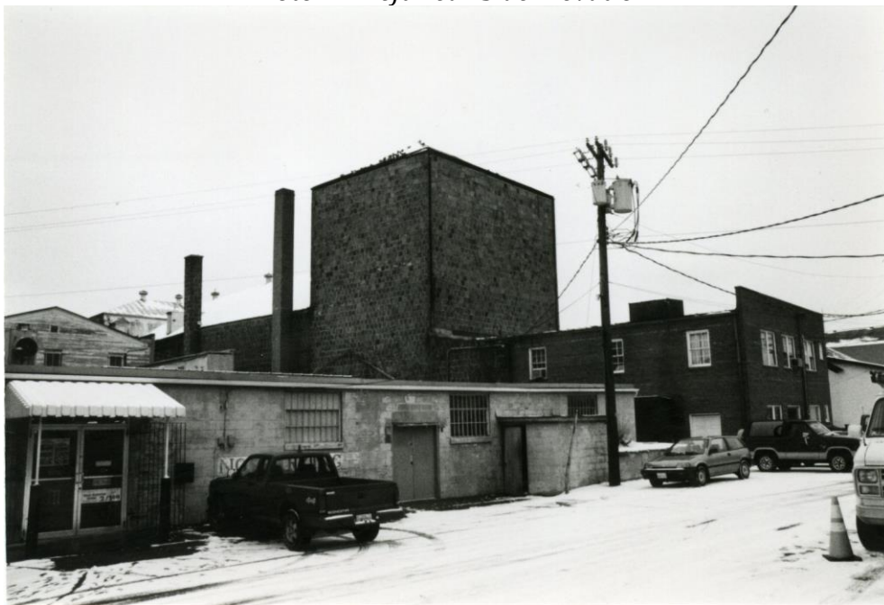
Photo 6 – Left Rear Side Elevation
