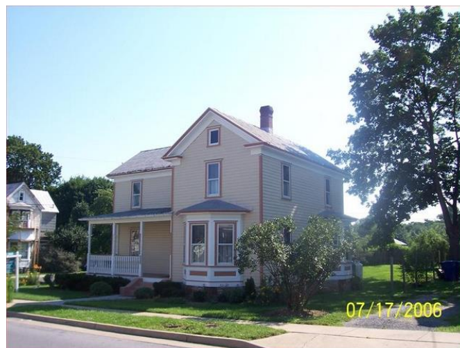
View of Front Right Elevation – 302 Blue Ridge Avenue
