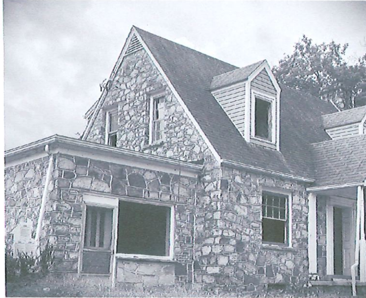
The original Main House of The Trellis before renovations.
