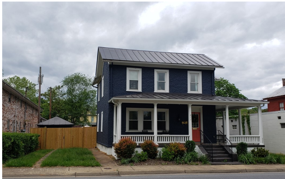
View of Front Elevation – 211 S. Royal Avenue
