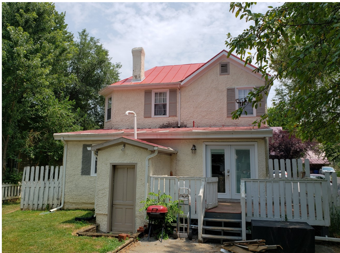
Photo 2 – view of rear building elevation – current view July 2023
