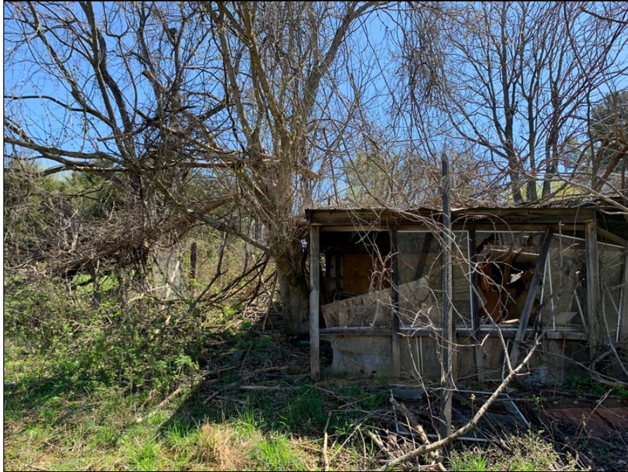
13 - Additional View of Storage Shed
