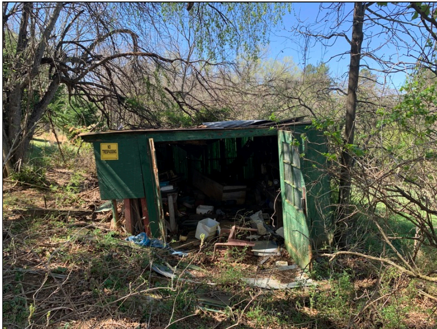
14 - View of Additional Storage Shed
