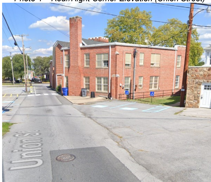
Photo 4 – Rear/Right Corner Elevation (Union Street)
