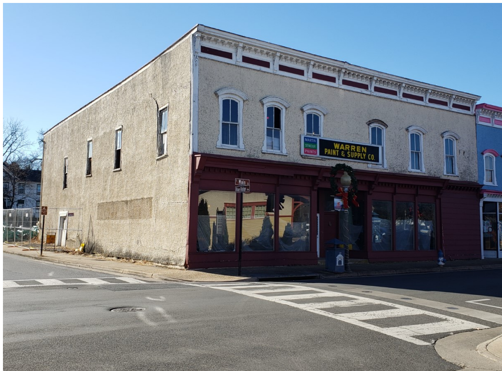
Photo 2 – Front & Left Side (Blue Ridge Avenue) Elevation
