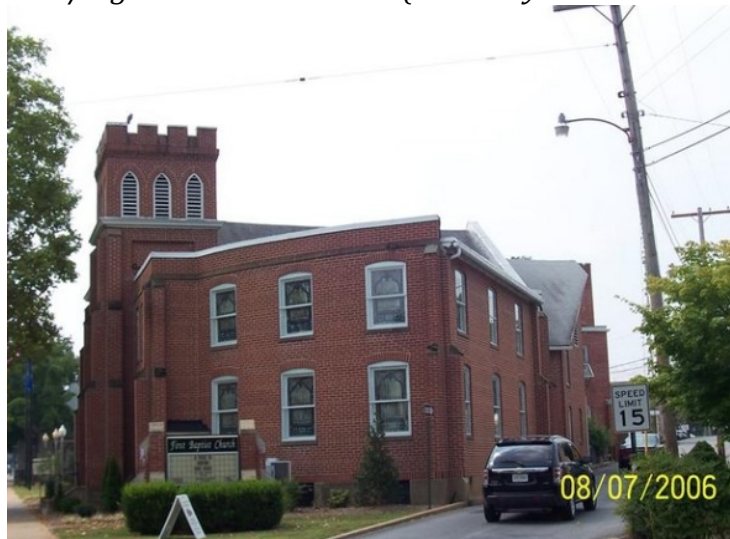
Photo 2 – Front/Right Corner Elevation (32 N. Royal Avenue & Union Street)
