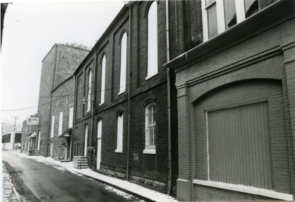
Photo 2 –Left Side Elevation (Church Street)
