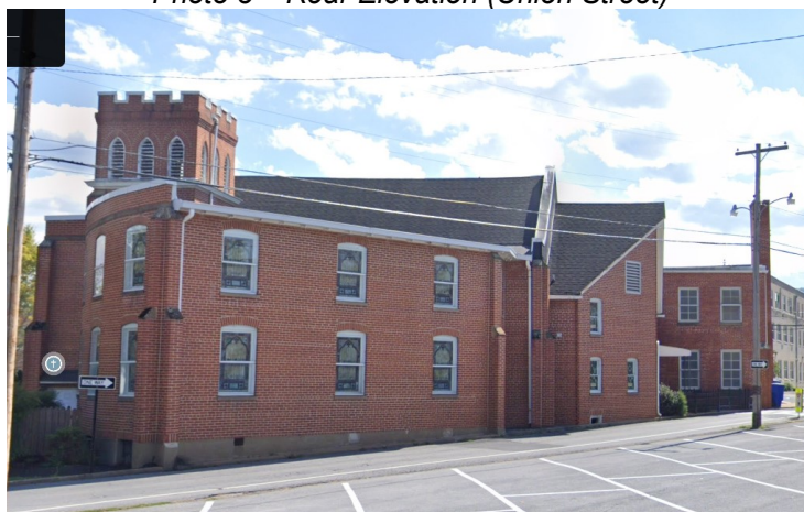
Photo 3 – Rear Elevation (Union Street)
