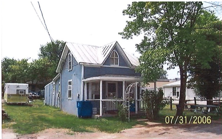
Previous Structure at 219 E. 7 th Street
