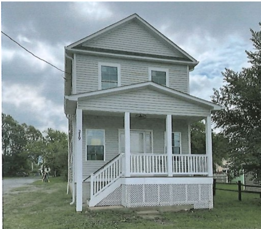
Existing Front Elevation (North) -219 E 7 th Street
