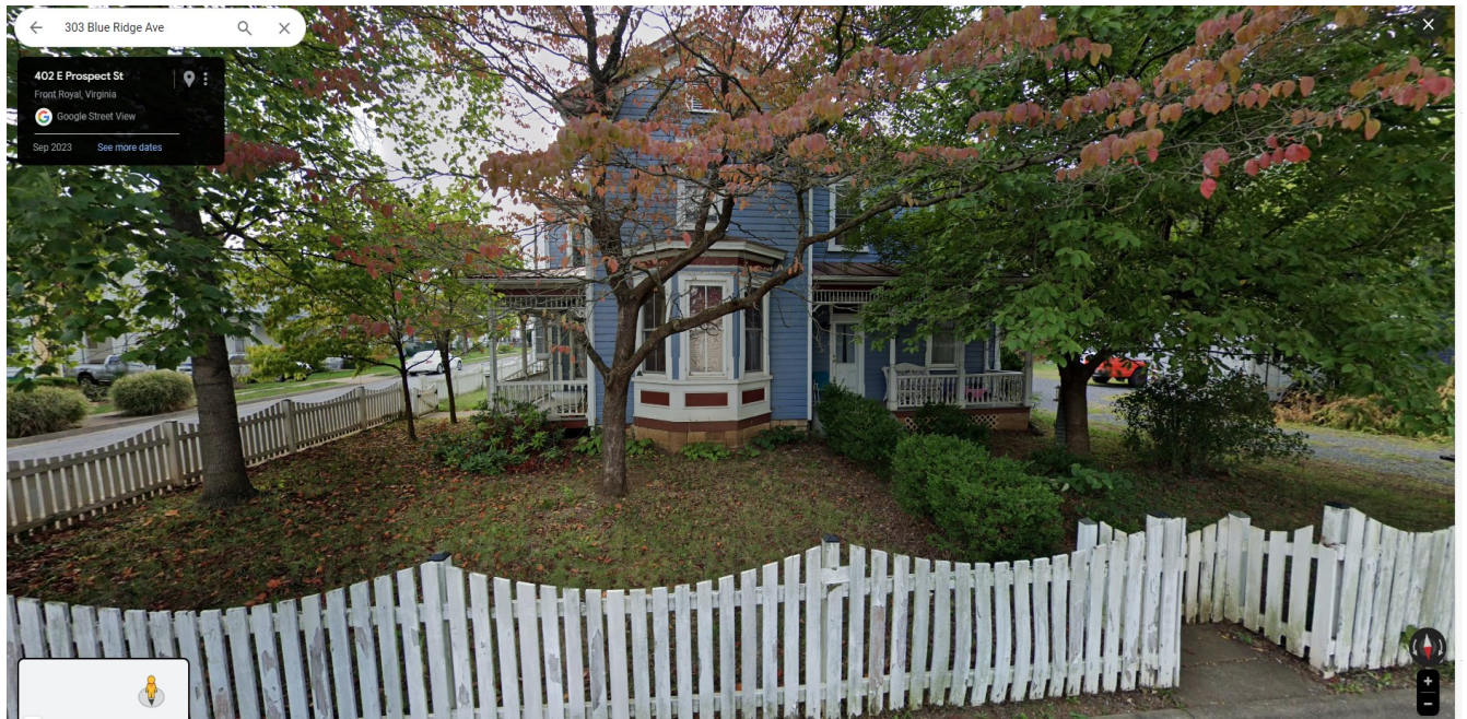
Photo 2 – View of Right Building Elevation (from E. Prospect Street) - Google Maps September 2023
