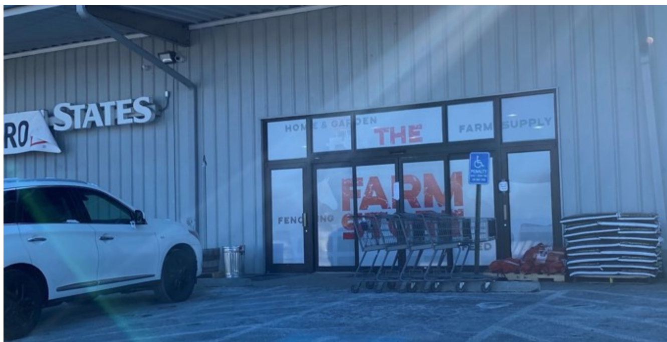
Photo 4 & 56 – Front Elevation of Existing Signage Already Installed at 50 Water Street
