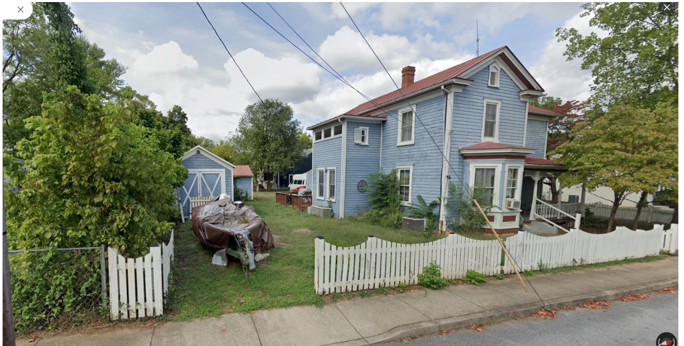
Photo 3 – View of Front Left Building Elevation – Google Maps – September 2023
