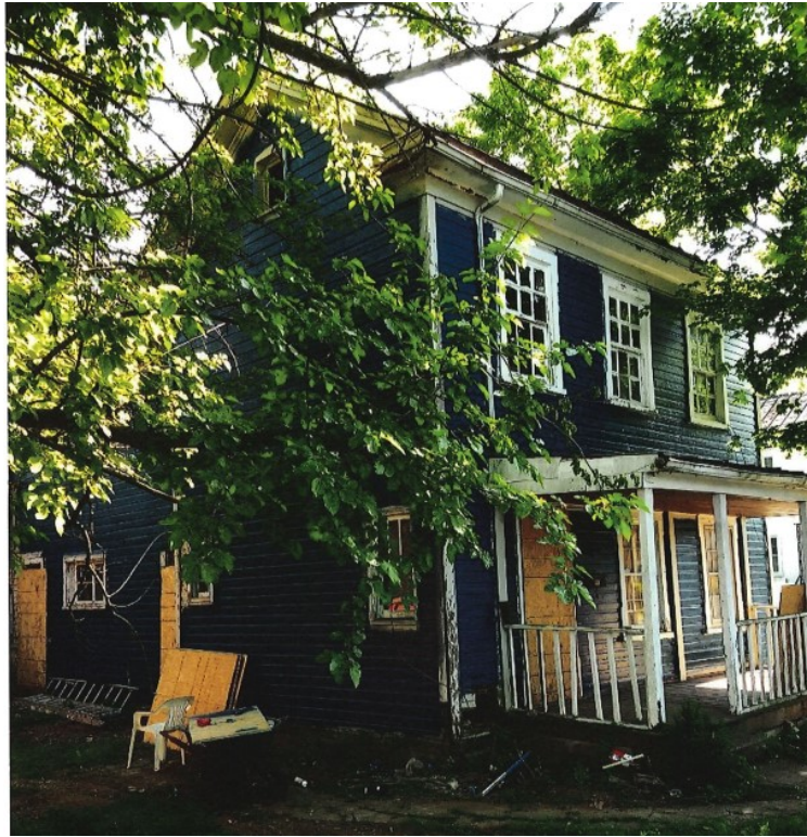
Photo 5 & 6 – view of blue painted wood siding before being replaced with a cream color vinyl siding (both done by applicant)
