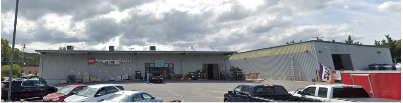
Photo 2 – View of Front Building Elevation - Google Maps July 2017
