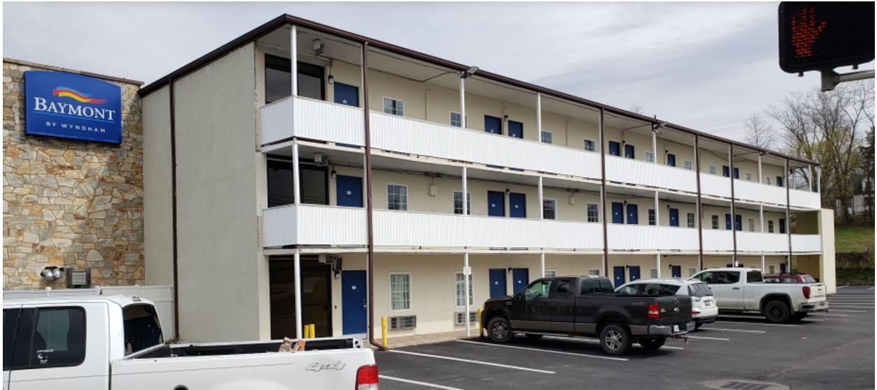
Rear Elevation – 10 S. Commerce Avenue
