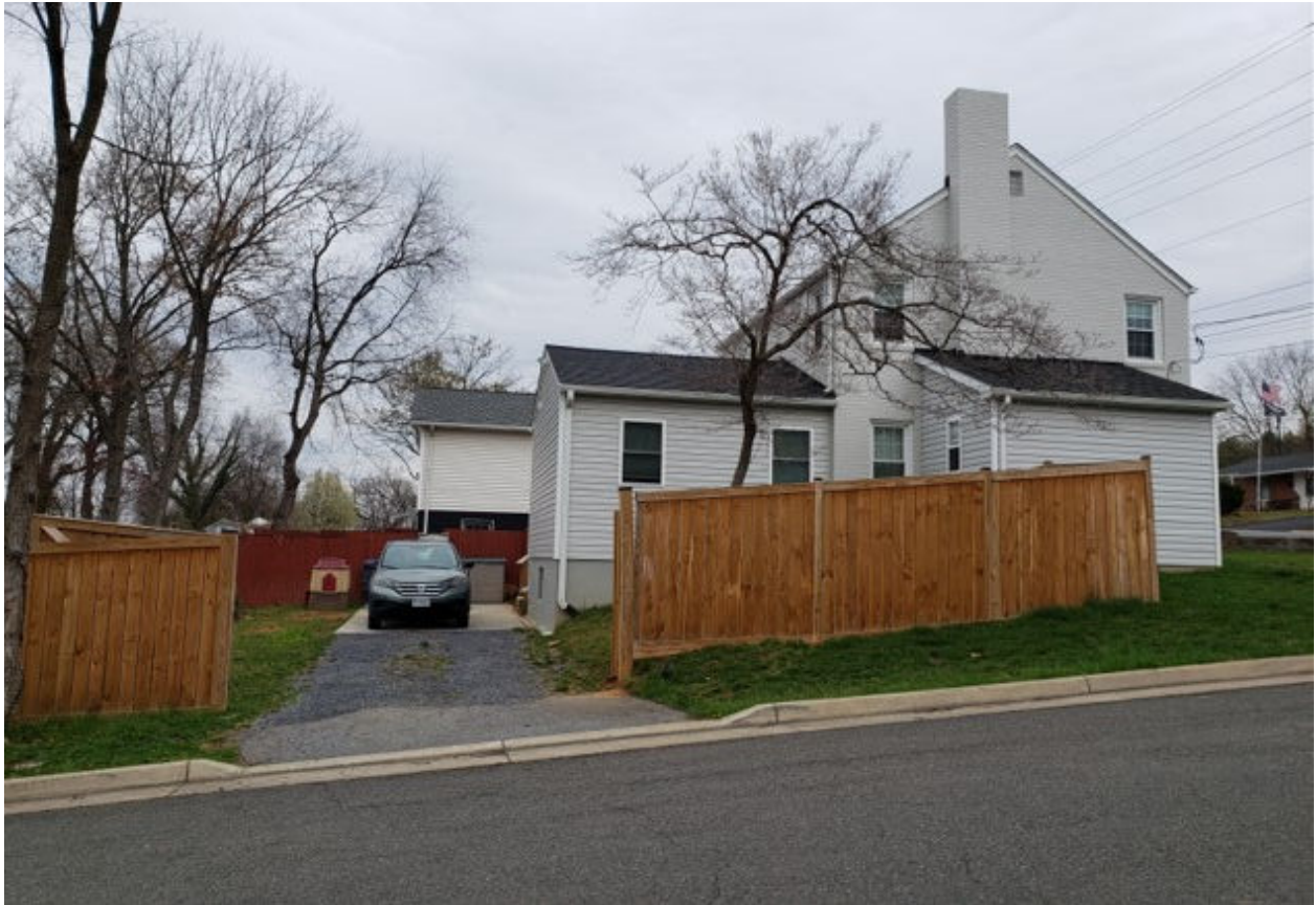
View of Left Elevation – 331 Kerfoot Avenue
