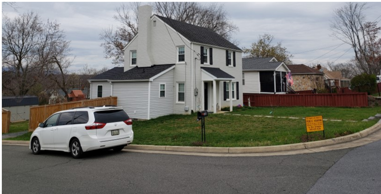
View of Front Left Elevation – 331 Kerfoot Avenue
