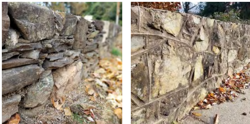
Figure 3-10: Dry stacked stone walls are a character-defining feature within the historic district (left). Some of the stone walls are laid with mortar, like this example that exhibits grapevine joints (right).
