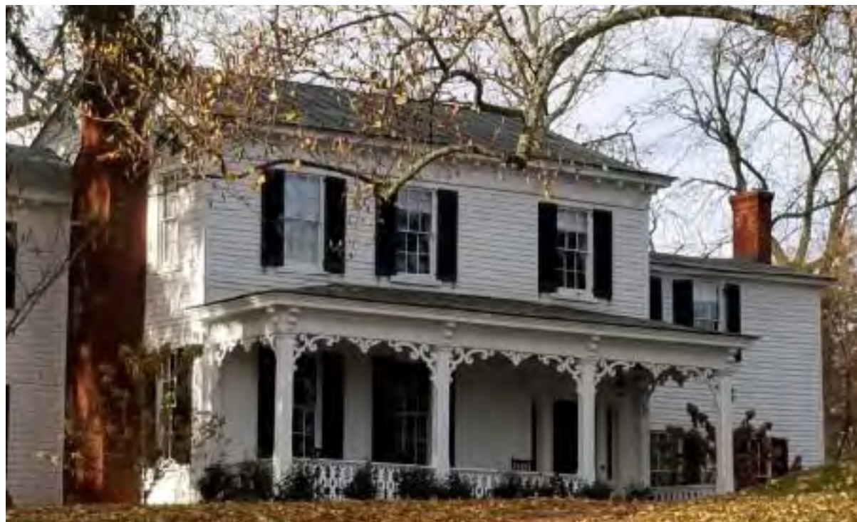
Figure 3-36: The porch on the excellent Italianate-style frame house has an intricate jigsaw balustrade, chamfered columns, and infrequent C-scroll brackets supporting the bracketed cornice.
