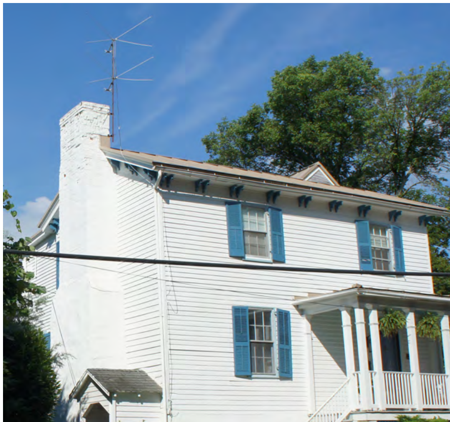
Figure 3-82: This antenna could be located in a more discrete location so as not to detract from the historic building.
