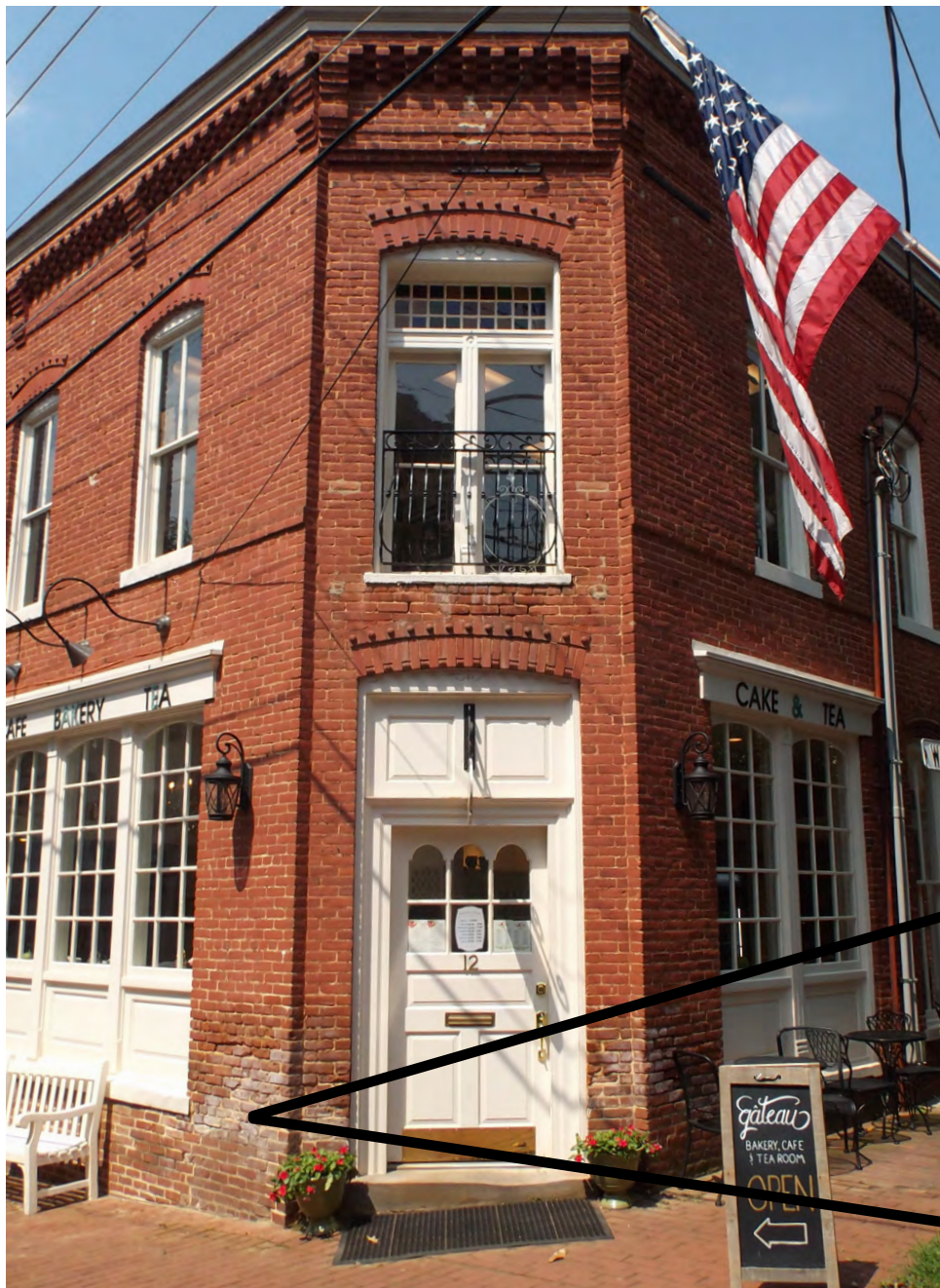
Figure 3-23: Salt efflorescence is a sign of perpetual moisture on masonry surfaces.
