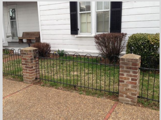
Illustration 18: Here is an example of a fence consisting of masonry posts.
