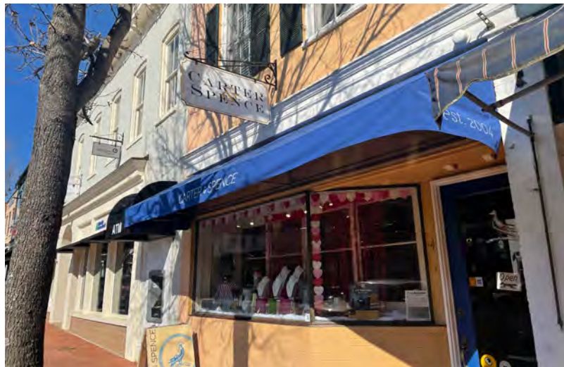
Figure 3-61: The awning at 41 Main Street is appropriately sized with subtle lettering to inform but not detract from the design.
