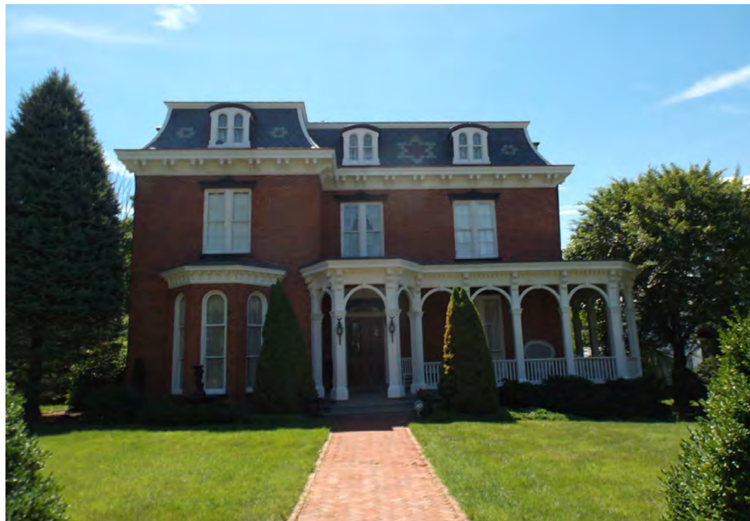
Figure 3-39: The Ullman House has a superb, patterned, polychromatic slate roof.
