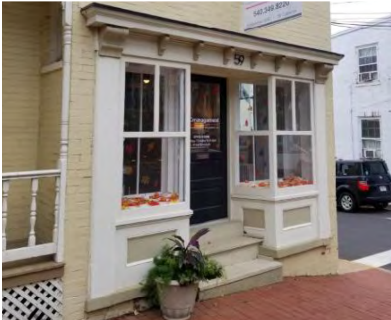
Figure 3-1: This storefront was added to a residential building during the district's period of significance. The non-original modification has gained significance in its own right.
