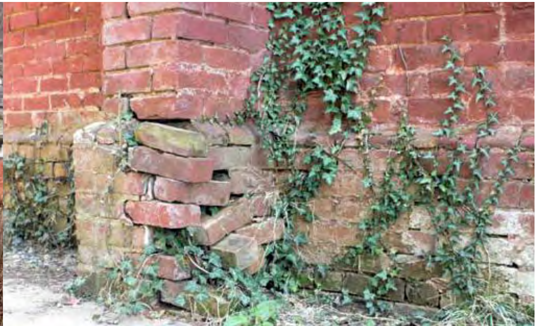
Figure 3-8: Do not allow ivy or other organic material to grow on a building or masonry wall. The vegetation will damage mortar joints, leading to structural damage as shown on the foundations of the first St. John's Catholic Church on Lee Street.
