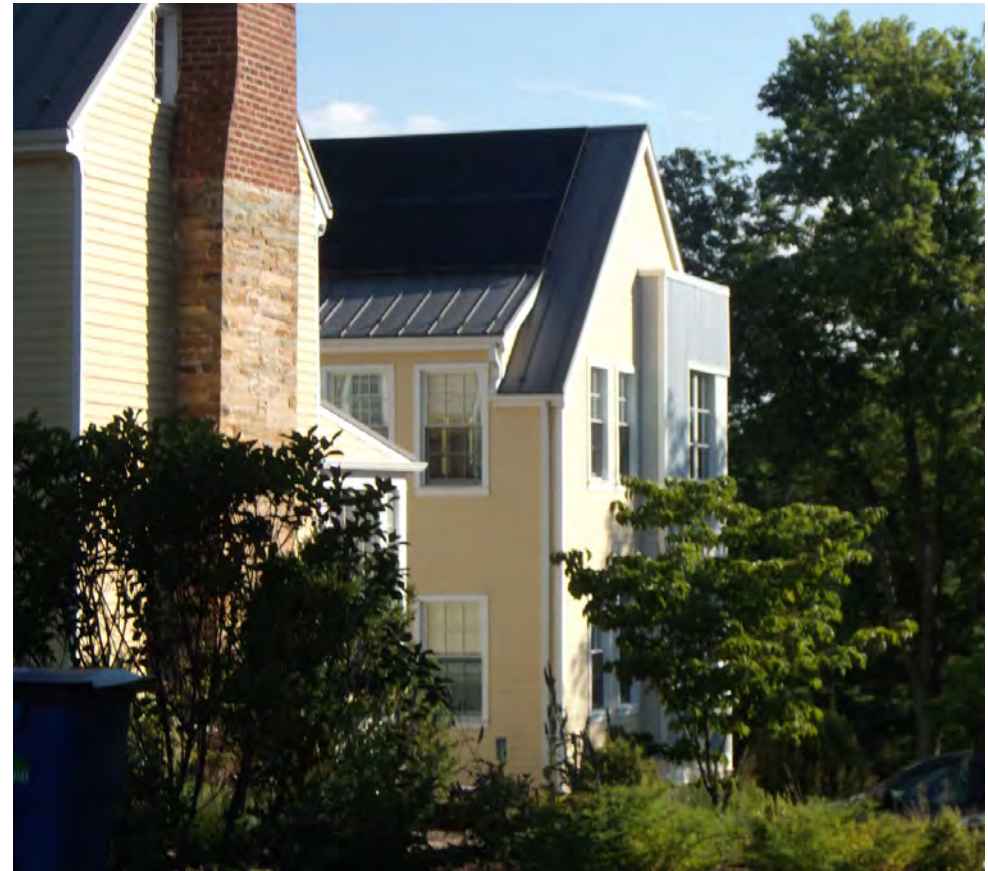
Figure 3-84: 45 Horner Street installed solar paneling on the new rear addition of the building preserving the integrity of the original structure while incorporating sustainable practices.
