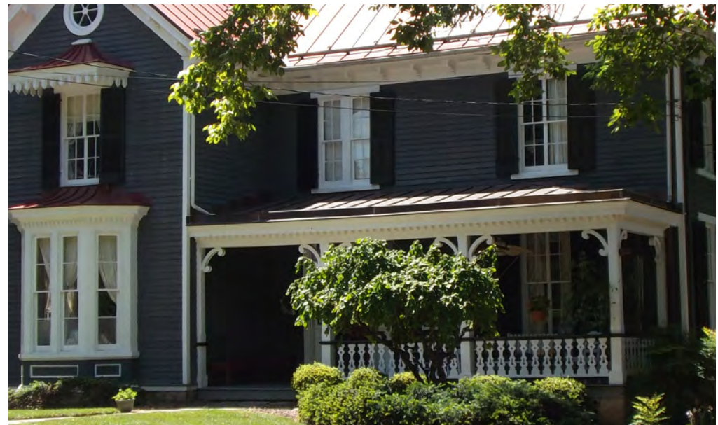
Figure 3-38: The porch on the excellent Italianate-style frame house at 178 Main Street has an intricate jigsaw balustrade, chamfered columns, and infrequent C-scroll brackets supporting the bracketed cornice.
