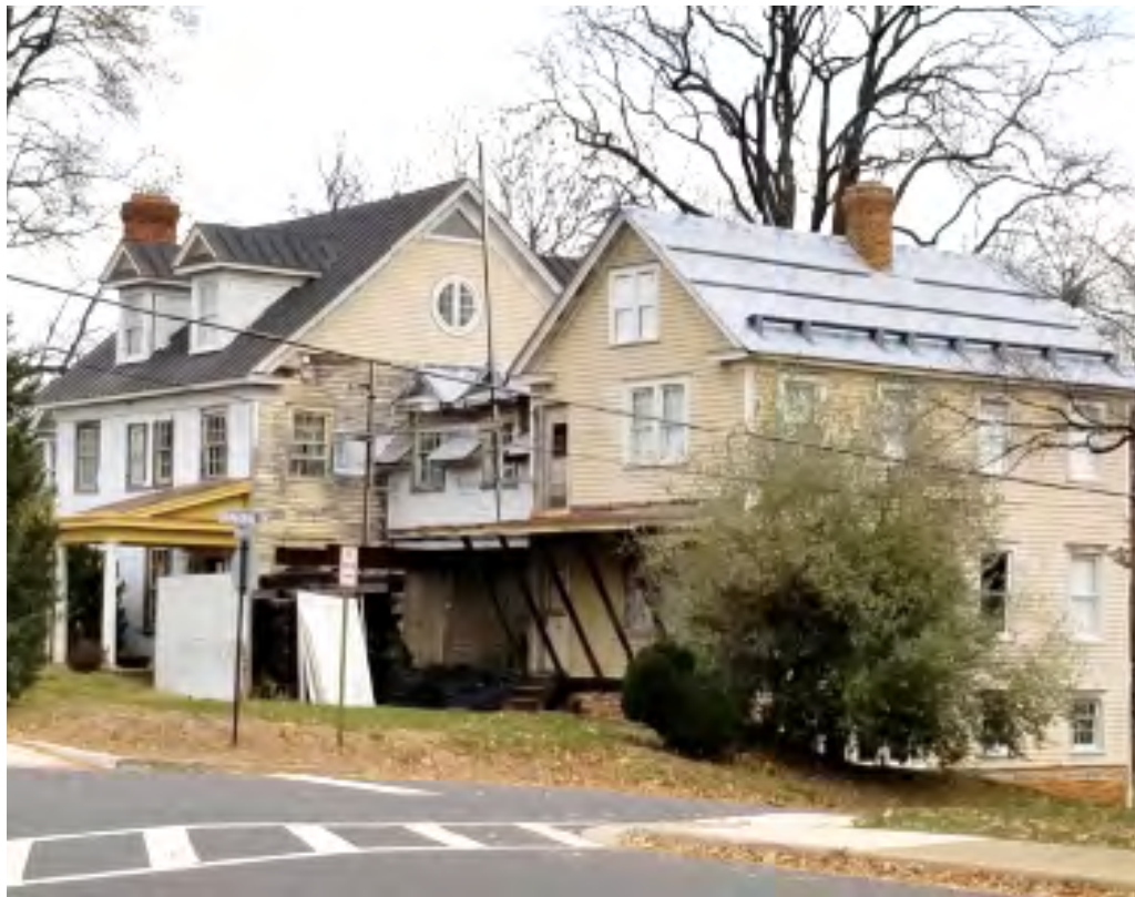
Figure 3-3: This building is utilizing temporary stabilization techniques to stabilize the front porch roof while the house is under construction. Temporary stabilization tactics should be approved on a temporary basis, with a definable end date for repairs to be completed.
