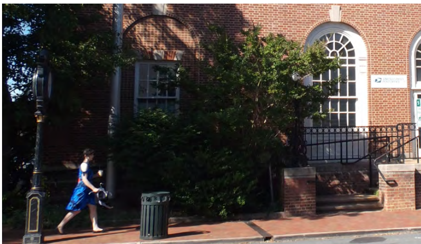
Figure 3-75: The ramp located at 53 Main Street is located on the side of the front entrance but is set back and landscaped to soften the impact on the streetscape.
