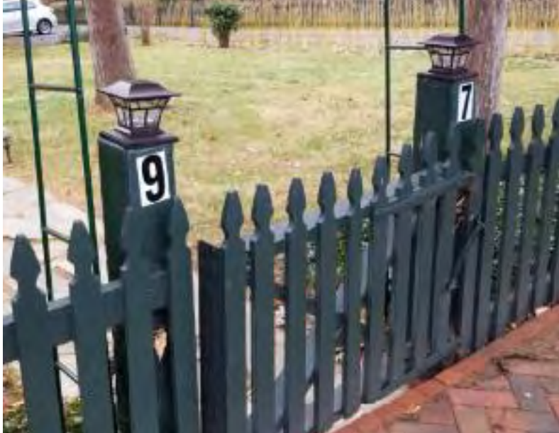
Figure 3-21: These solar lights are small and discrete and can be removed easily if desired. They illuminate the gateway while keeping light pollution to a minimum. A more permanent solution would also be appropriate here.
