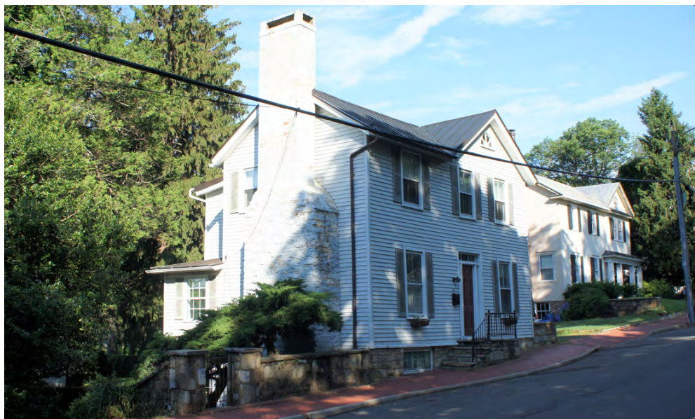
Figure 3-40: 84 Winchester has a heavy chimney with lower corbels aligning with the dense structural emphasis of Federal architecture.
