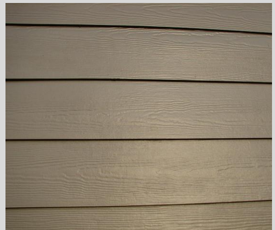
Illustration 22 : Some sidings may be appropriate for a renovation project when it is unfeasible to restore wood siding. Above is picture of hardiplank siding, which is difficult to distinguish from wood.
