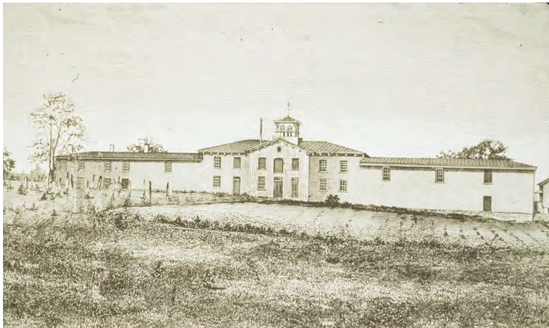
Figure 1-11: The main house at Monterosa was initially constructed ca. 1847 for the residence of William (Extra Billy) Smith, former Governor of Virginia, then heavily altered ca. 1865 for James K. Maddux, leader in the establishment of the Warrenton Hunt. This property was individually listed on the National Register of Historic Places in 1991 as the Governor William "Extra Billy" Smith Stables and Slaves Quarters (156-0020). Image from the VDHR VCRIS database.
