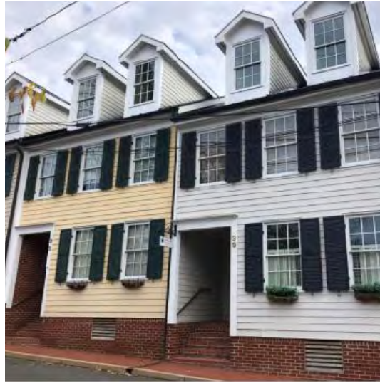
Figure 3-100: These modern row-houses are situated within the historic district and blend seamlessly with their environment. The houses reflect their surroundings, yet are differentiated through an innovative, recessed, entryway; oversized dormers; and modern materials.
