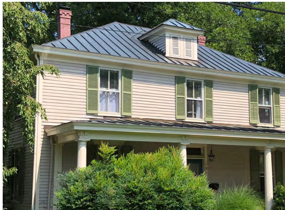
Figure 3-41: The dual chimneys at 181 High Street add to the symmetry of the building which is a notable element of four-square architecture.
