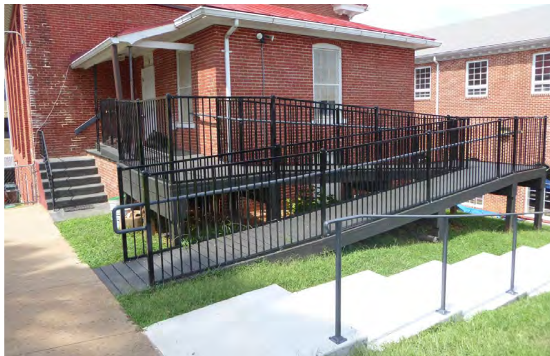
Figure 3-76: The ramp at 39 Alexandria Pike is located at the rear of the property only visible from a municipal parking lot minimizing the impact on the historic streetscape of Alexandria Pike.
