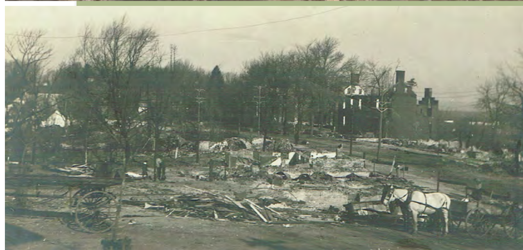
Figure 1-14: Various images of the damage caused by the 1909 fire on the western edge of now Old Town Warrenton. Image from the Fauquier County Historical Society.
