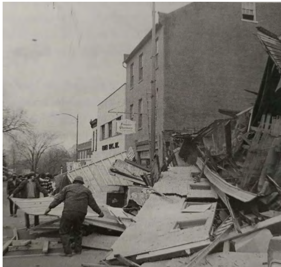
Figure 3-104: 21 Main Street had previously been three separate structures before coming together to become Town Hall. This is a picture of the facade collapse during the building demolition in September, 1974. Image from the Warrenton, Virginia book by Toler, Shepherd, & Power.
