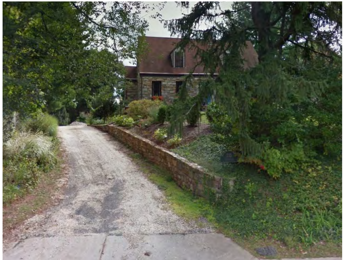
Figure 3-13: This driveway was cut through the hillside and retained with a stone wall. Whether original to the house or added at a later date—the appropriate design minimally affects the integrity of the house.
