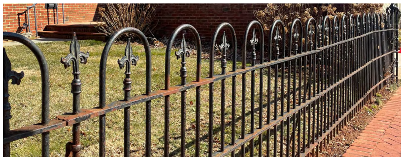
Figure 3-9: Cast-iron fences are common in the historic district.
