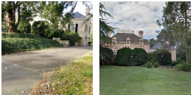
Figure 3-12: This driveway (left) was added to the side of a residential property by cutting into the hillside. The gradual grade change is disguised with ground cover and is minimally visible from the front of the building (right).
