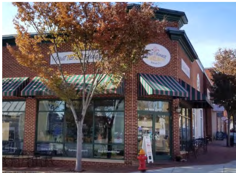
Figure 3-33: This awnings on this commercial building are appropriate for Warrenton's commercial downtown.
