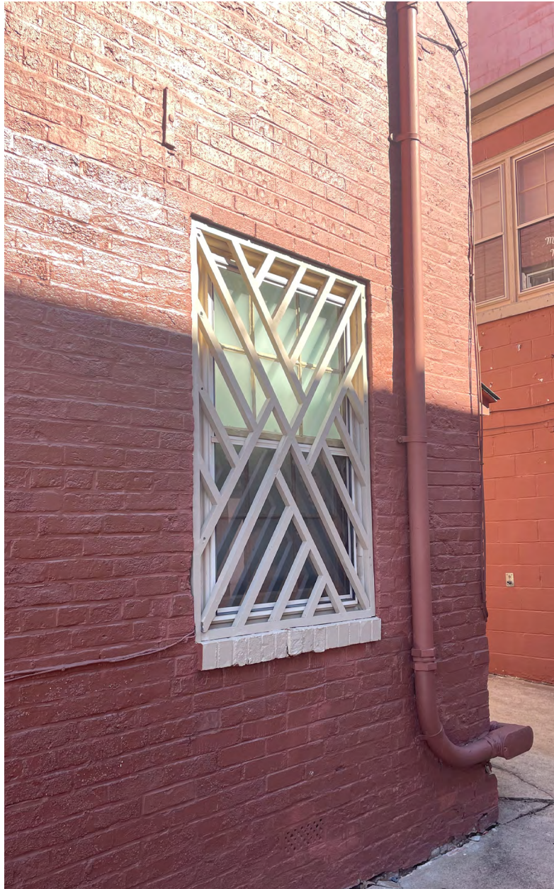
Figure 3-74: This wood screen at the rear of 88 Main Street adds an additional decorative element while providing the necessary security and energy efficiency.
