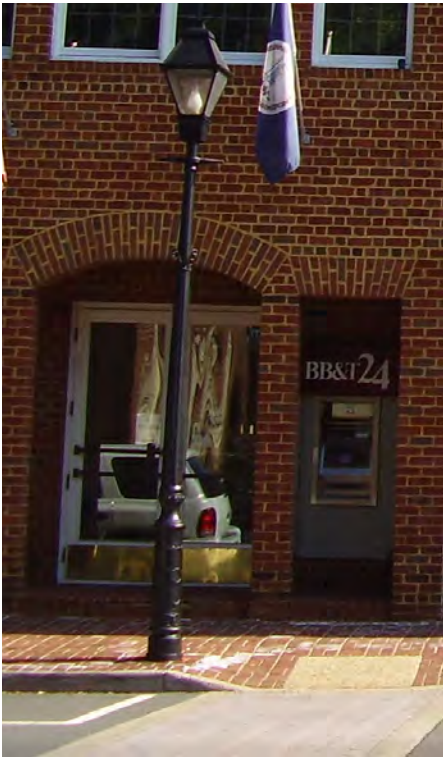
Figure 3-79: 21 Main Street ATM before it was removed.
