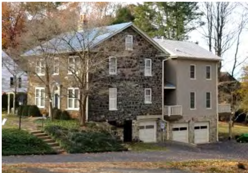
Figure 3-103: This photograph illustrates a successful addition to the rear of a historic residential property. The addition is clearly differentiated from and subordinate to the original house, yet also shows similar massing, scale, rhythm of openings, roof line, and color scheme.
