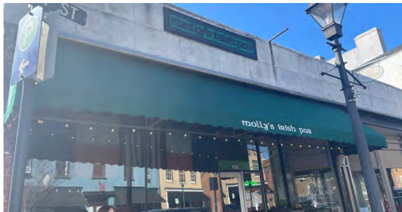
Figure 3-62: The 36 Main Street awning sign does cover or obscure the architectural details on the structure.
