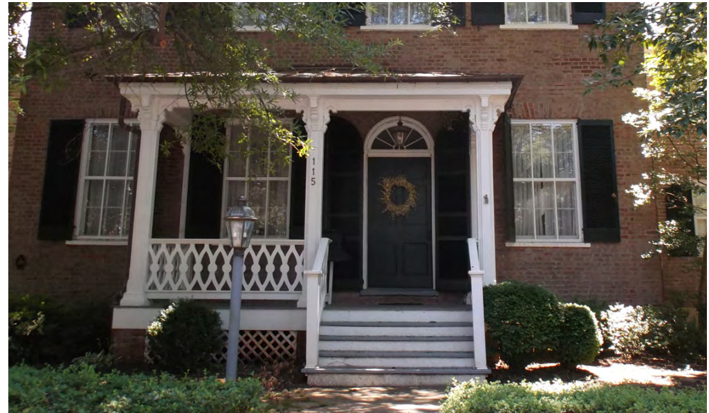
Figure 3-37: This one-story, two-bay porch with an intricate scroll-sawn balustrade was added to the Federal-style H. Clay Ward House at 115 Culpeper Street in the late nineteenth century.
