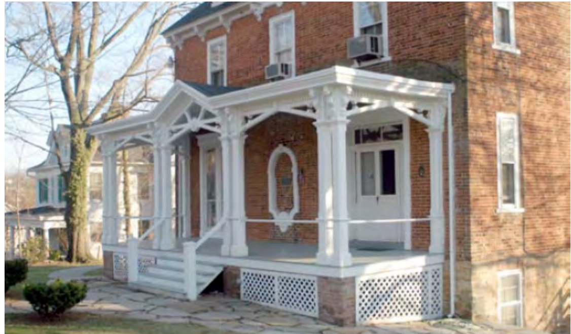
Figure 3-2: This richly-detailed Italianate-style porch was added to the Federal-style, circa 1830 Robert Brent House at 114 Lee Street, during General William H.F. Payne's 1866-1901 ownership.
