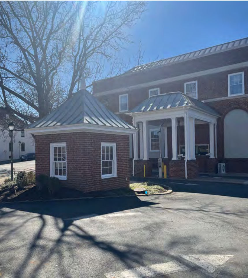
Figure 3-80: 10 Courthouse Square is not a traditional ATM but incorporates banking window needs into the existing structures with compatible detailing to complement the architecture.
