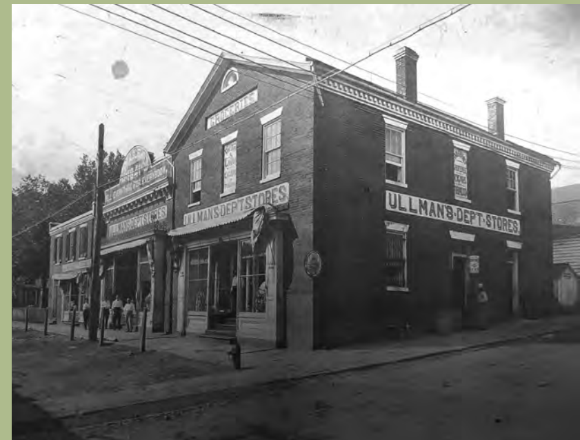
Figure 1-10: The Ullman department store complex at 49-53 Lee Street started operation in 1852 by Abraham Rindsburg and his son, Adolph Rindsburg. Image from the Fauquier County Historical Society.
