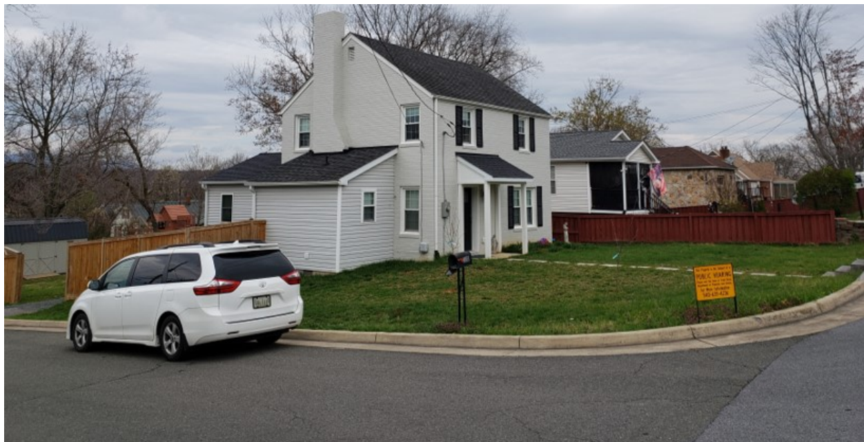
View of Front Left Elevation – 331 Kerfoot Avenue
