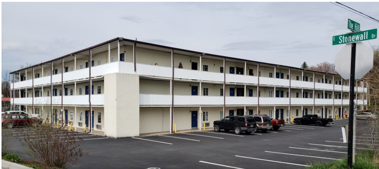
Right-Rear Elevation – 10 S. Commerce Avenue
