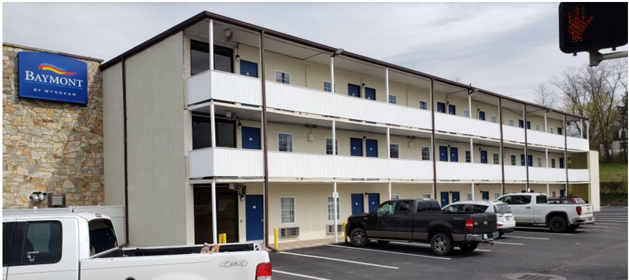
Rear Elevation – 10 S. Commerce Avenue
