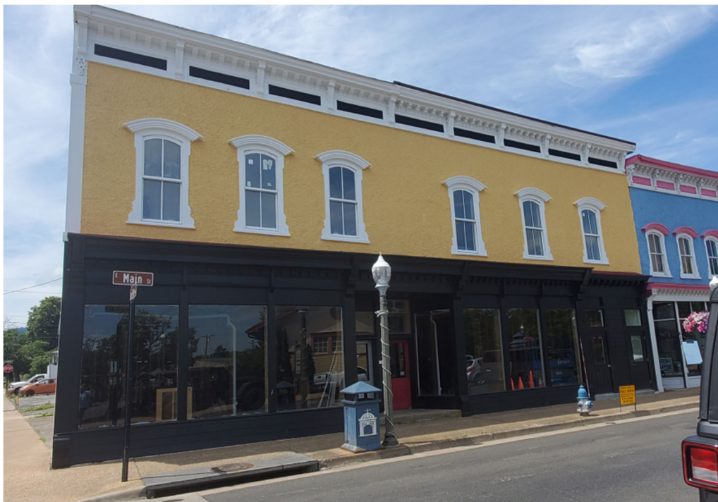
View of Front Left Elevation – 415 E. Main Street
