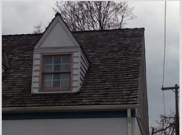
Illustration 6: Metal, slate and wood shingle roofs are compatible with the original architecture of the buildings in the historic district. Above is a picture of a roof with cedar shingles.
