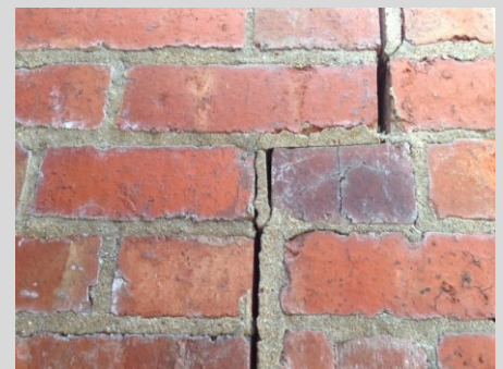
Illustration 14: Proper maintenance of masonry will help prevent expensive repairs in the future.
