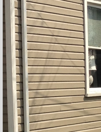
Illustration 20: Rather than covering a building with vinyl, it is preferred that the natural wood be maintained. Above is a good example of maintained wood.
