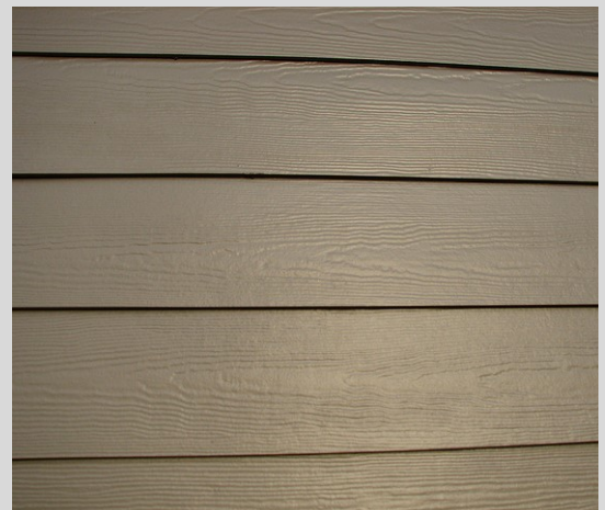
Illustration 22 : Some sidings may be appropriate for a renovation project when it is unfeasible to restore wood siding. Above is picture of hardiplank siding, which is difficult to distinguish from wood.
