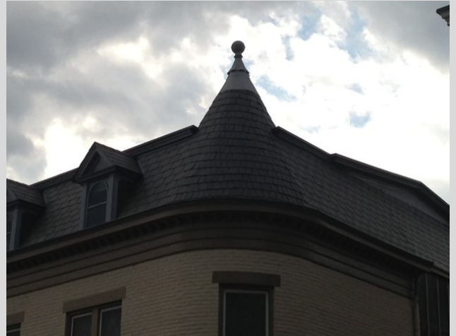
Illustration 7: Slate roofing, such as that shown above, is among the most durable roofing material.
