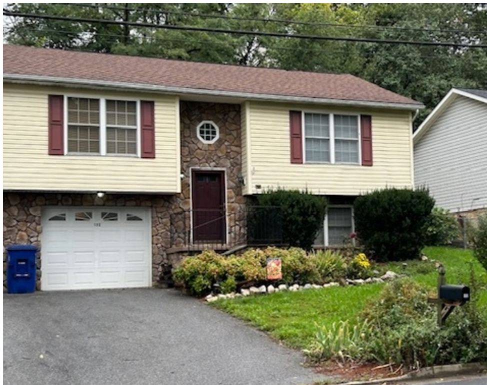
View of Front Elevation – 132 W. Criser Road
