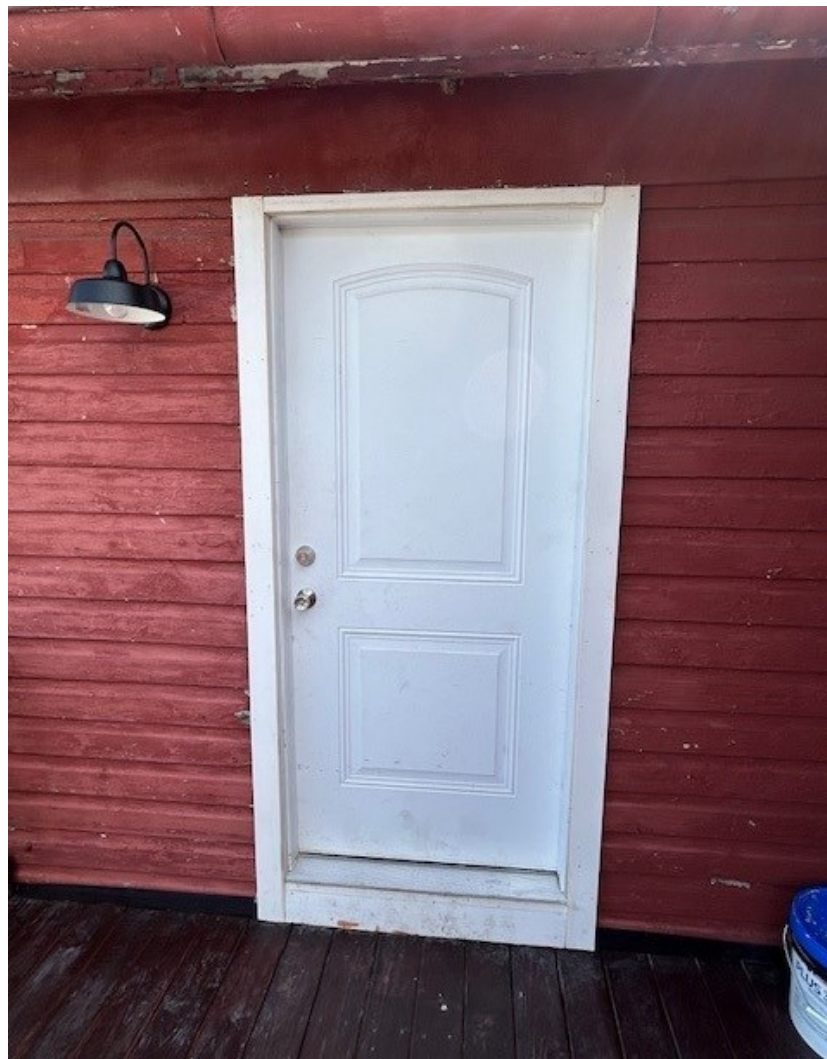
Rear Elevation Removed Existing Window and Replaced With A Door - 207 S. Royal Avenue
