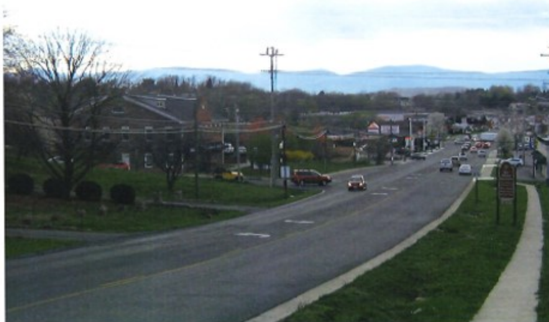
Photograph 2. John Marshall Highway at Royal Lane (View facing west)
