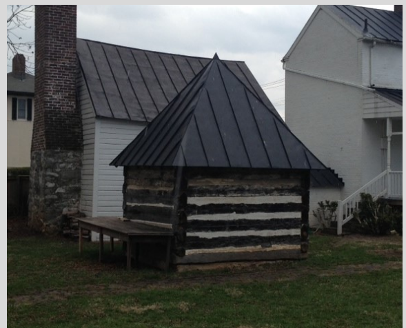
Illustration 16: Accessory buildings can also be significant assets of the historic district.
