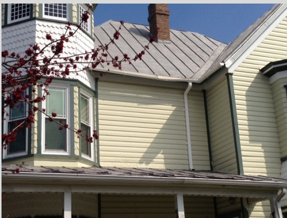
Illustration 21 : Above is another example of a house with a maintained wood exterior.
