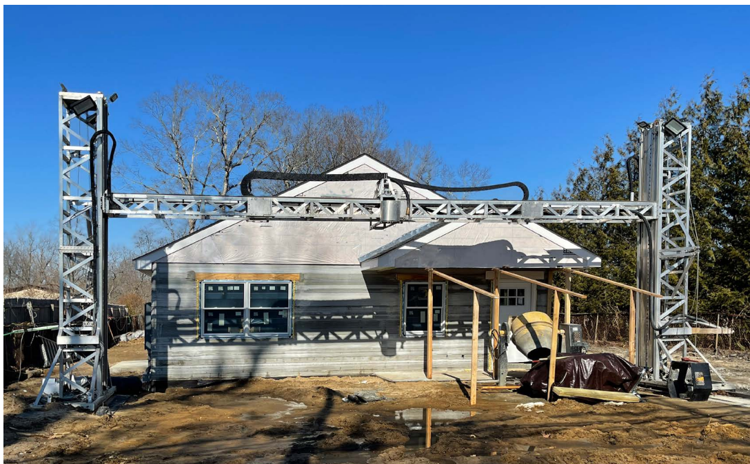
A 3D-printed house under construction in Riverhead, New York (Credit: futurewalk/iStock Unreleased)
