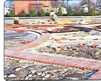
Brick work on around the Gazebo
