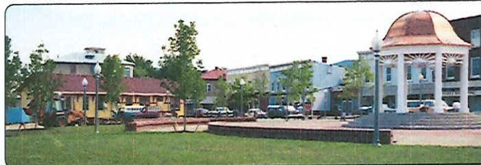
Final Stages of the Plaza
