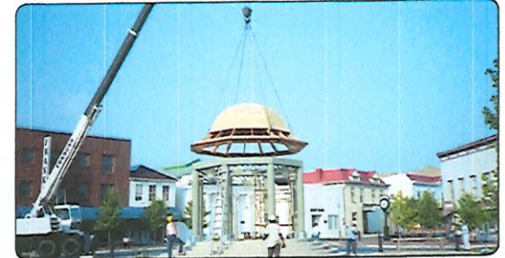
Hoisting the Dome atop the Gazebo
