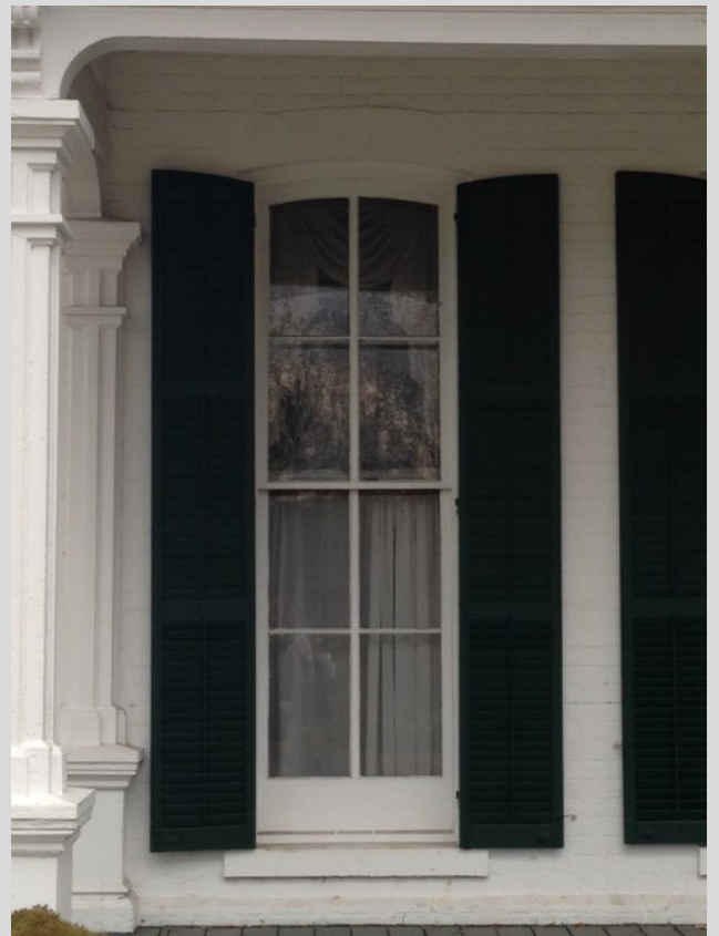
Illustration 12: Repair original windows instead of purchasing new windows.
