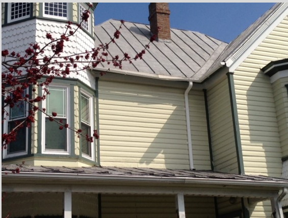
Illustration 21 : Above is another example of a house with a maintained wood exterior.
