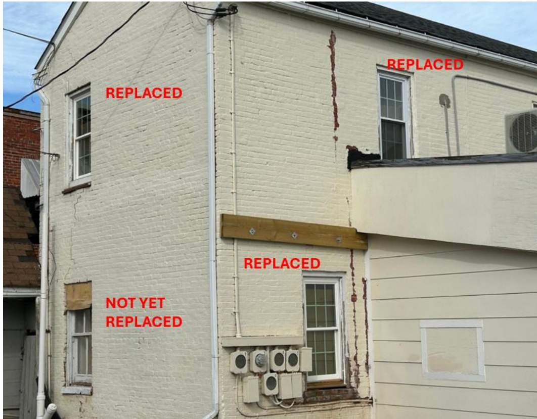
Photo 4 – Left Rear Elevation of 507 E. Main Street – May 3, 2025
