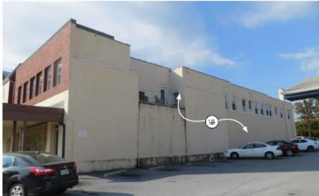
EXISTING SIDE FACADE
