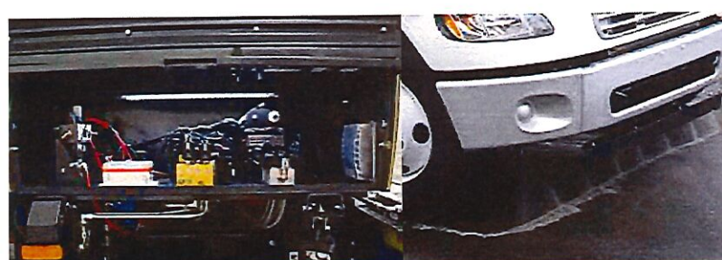
Accessible systems locker with LED service light.
