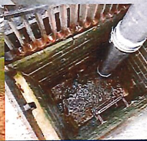
Powerboom option cleaning catch basin.
