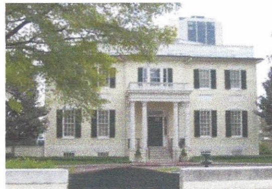
JTS was selected by DGS to oversee renovations at the Governor's Mansion.
