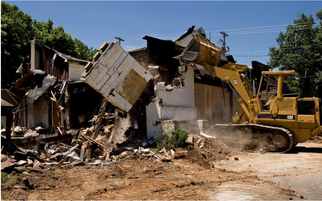
Picture (the old lodge being demolished after 2015 fire destruction)
