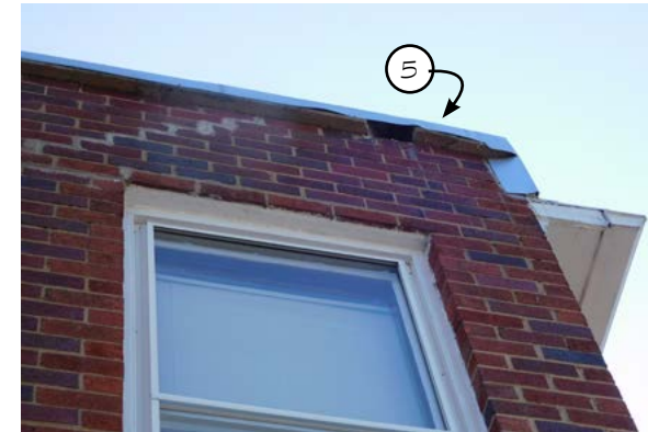
3 EXISTING PARAPET CAP NOT TO SCALE
