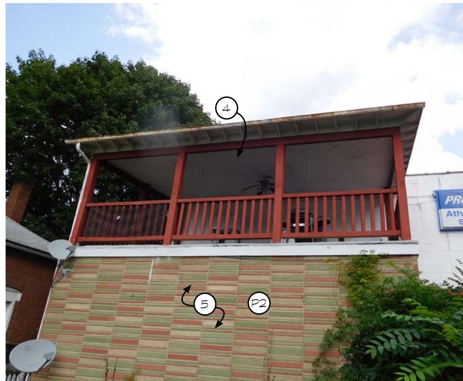
4 EXISTING SIDE FACADE NOT TO SCALE
