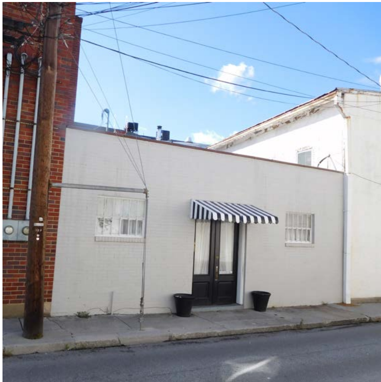
1 EXISTING CLOUD STREET FACADE NOT TO SCALE
