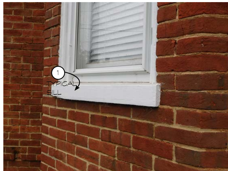
5 TYPICAL WINDOW SILL NOT TO SCALE
