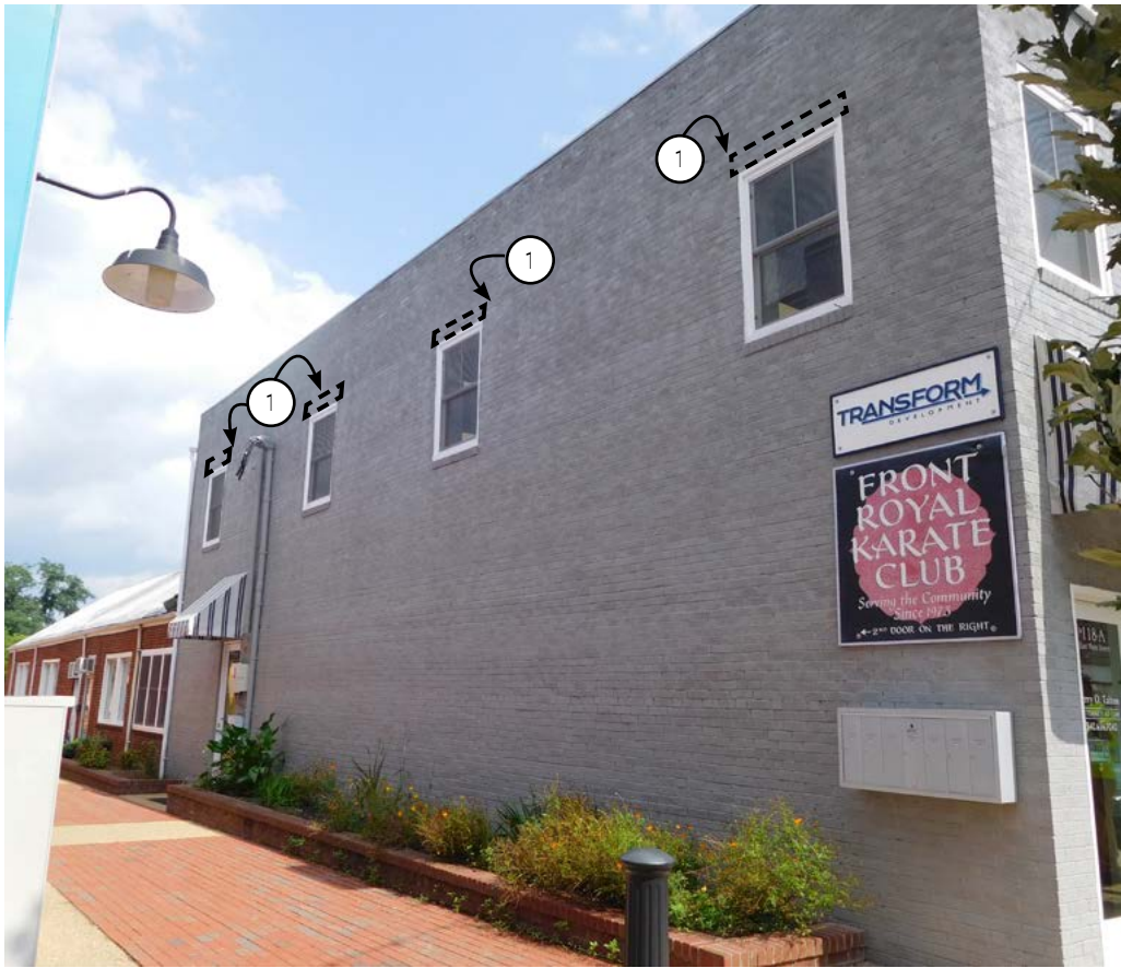
2 EXISTING SIDE FACADE NOT TO SCALE
