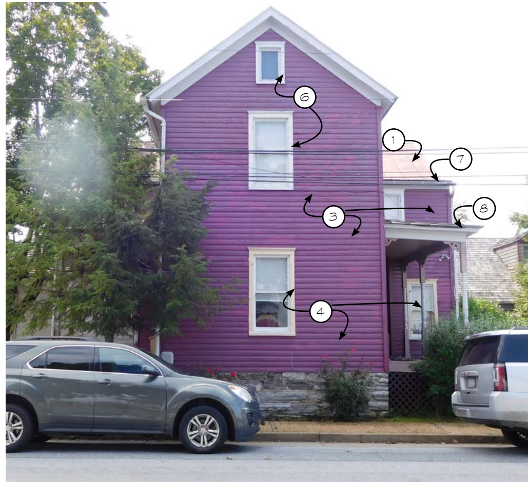
3 EXISTING CRESCENT STREET FACADE NOT TO SCALE
