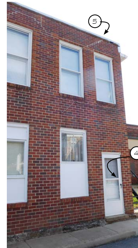
6 EXISTING SIDE FACADE NOT TO SCALE
