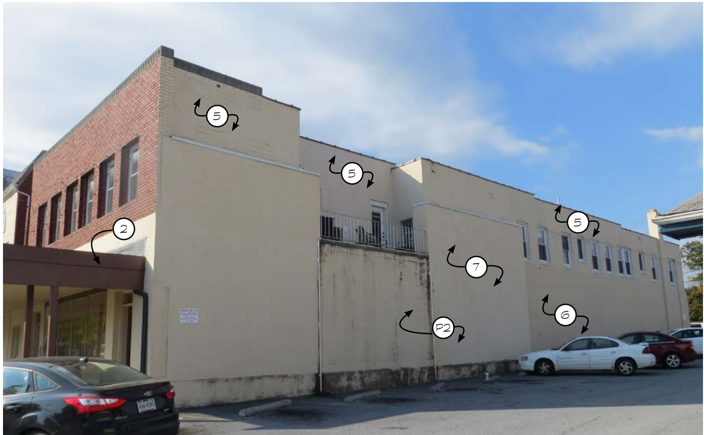
2 EXISTING SIDE FACADE NOT TO SCALE
