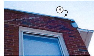
③ EXISTING PARAPET CAP NOT TO SCALE
